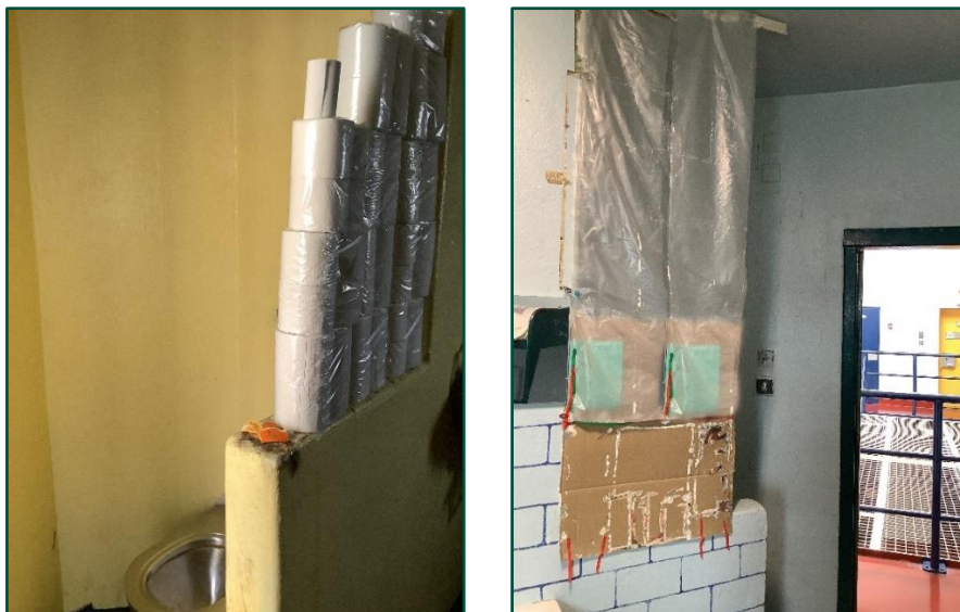
Figure 2: In-Cell Sanitary Facilities
